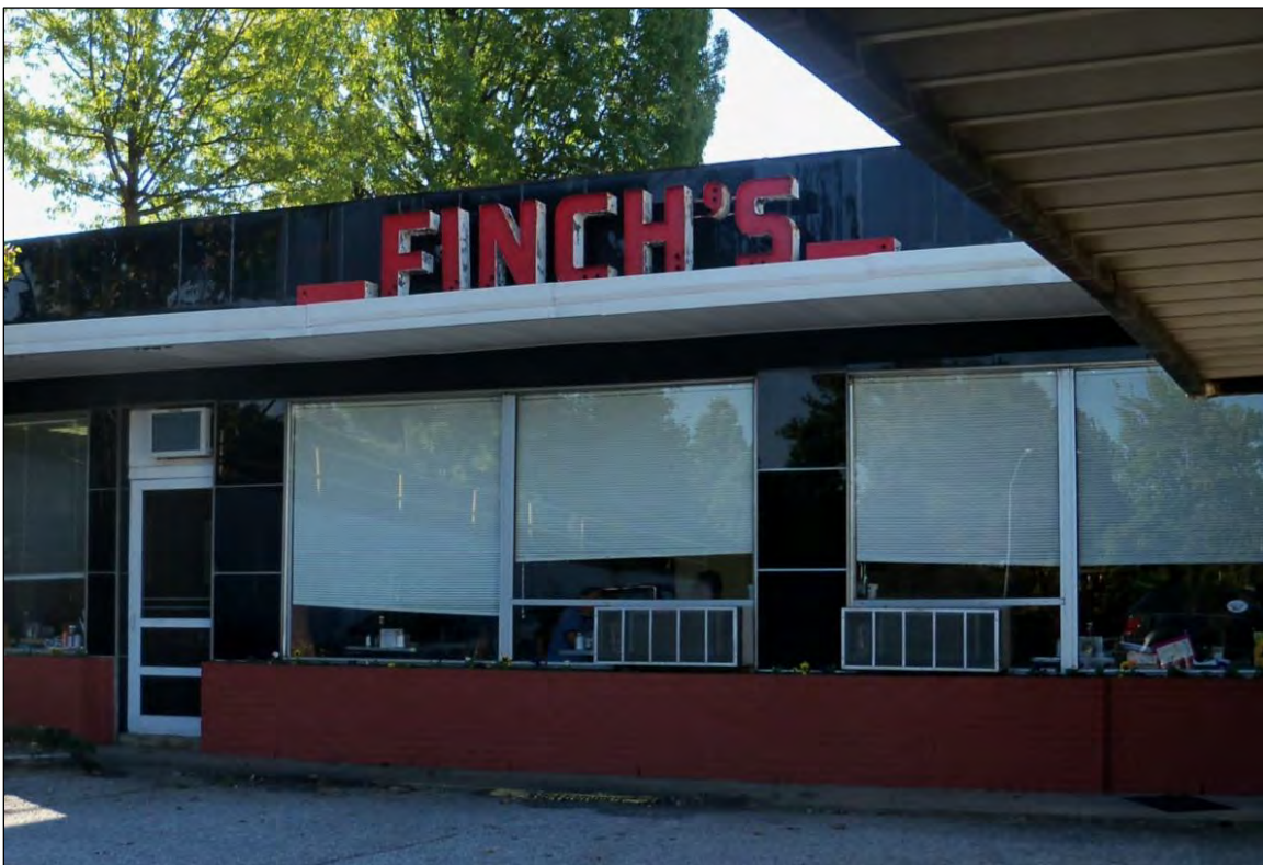
Photo 11: Detail of Façade and Sign, North Elevation of Finch's Restaurant.
