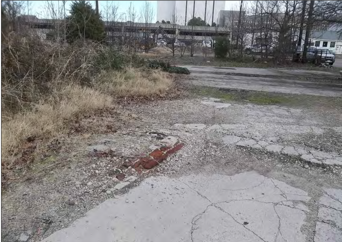
Photo 26: View of Various Materials and Foundations On-Site, Looking East.
