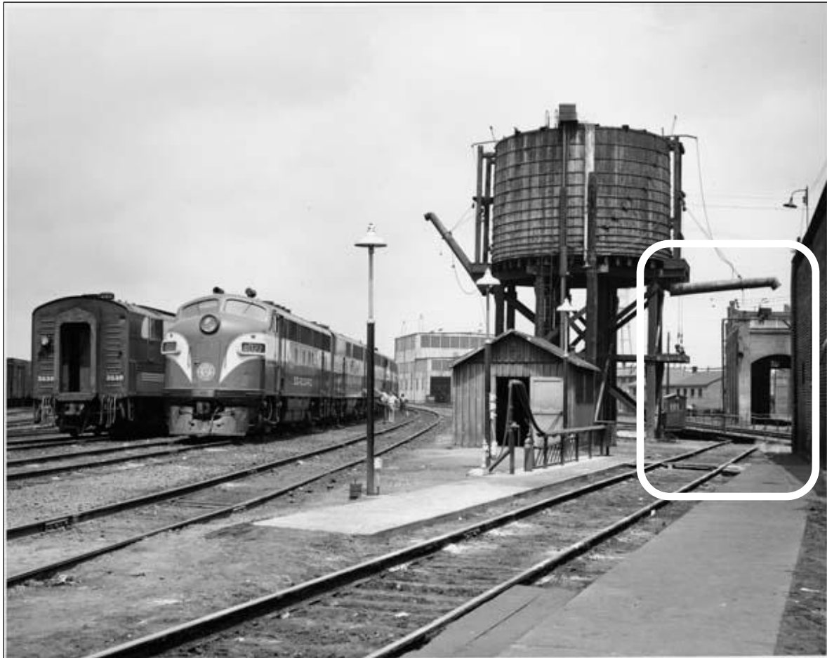
Photo 25: “In railroad yard, water tower in foreground; shop building in background...” (Lewis P. Watson Collection, Olivia Raney Local History Library). The east end of the roundhouse, the turntable, and its motor house are visible in this circa-1940s image.
