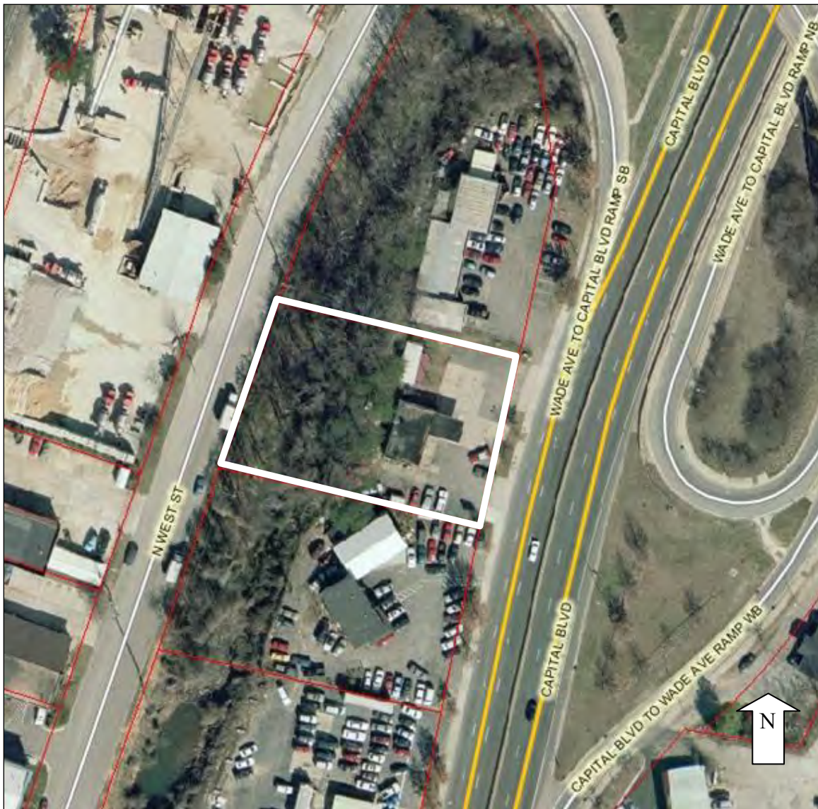
Figure 9: Map of Gulf Gas Station (WA 7363) NHRP Boundaries and Current Tax Parcel, Highlighted in White (City of Raleigh and Wake County imaps 2012).
