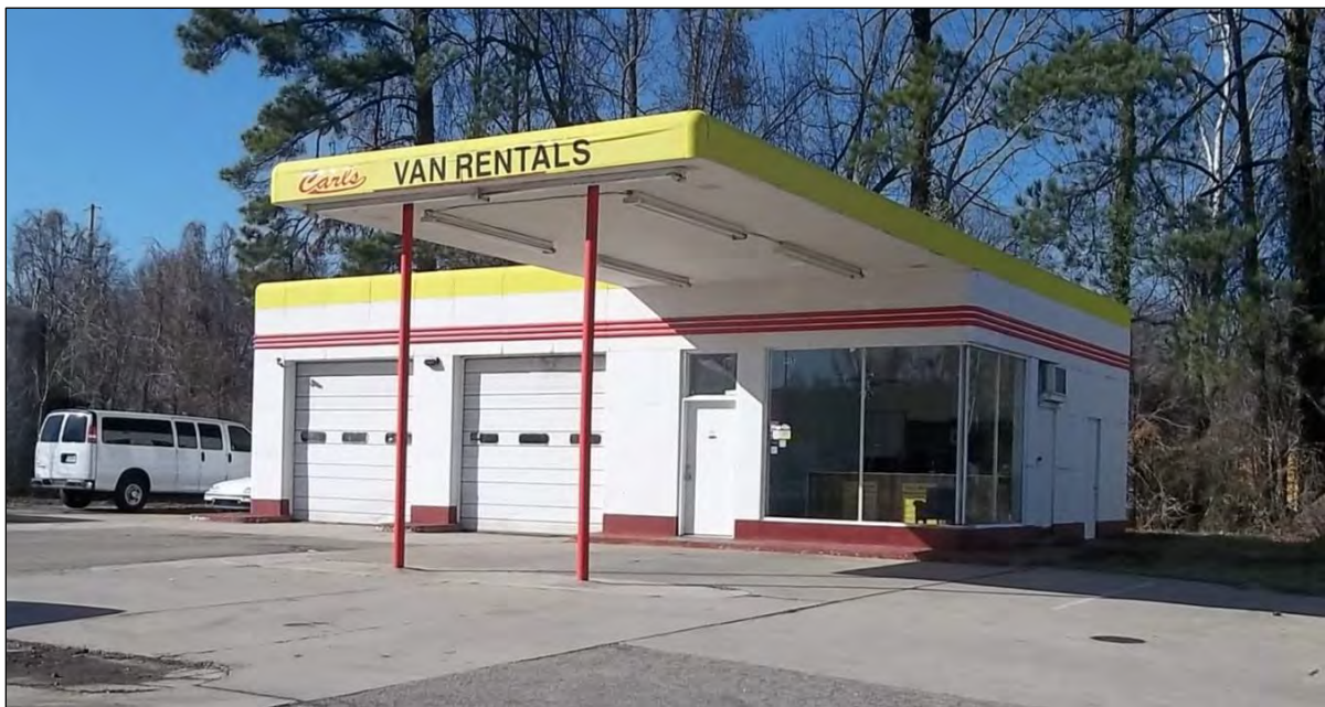
Photo 4: Northeast Oblique, Gulf Gas Station (WA 7363).
