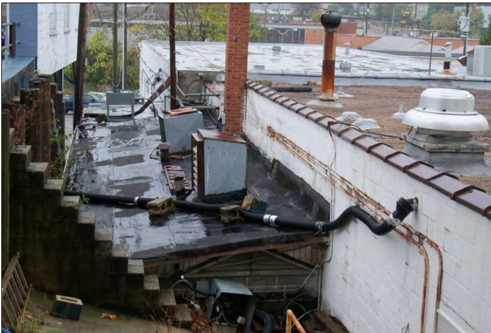
Photo 13: View of Rear Lean-to Addition, Looking West from Capital Boulevard Sidewalk.
