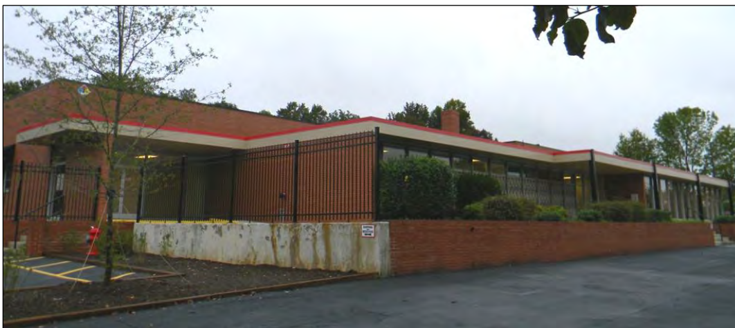
Photo 2: View of East Elevation, Noland Plumbing Company (WA 7126) Looking Northwest.
