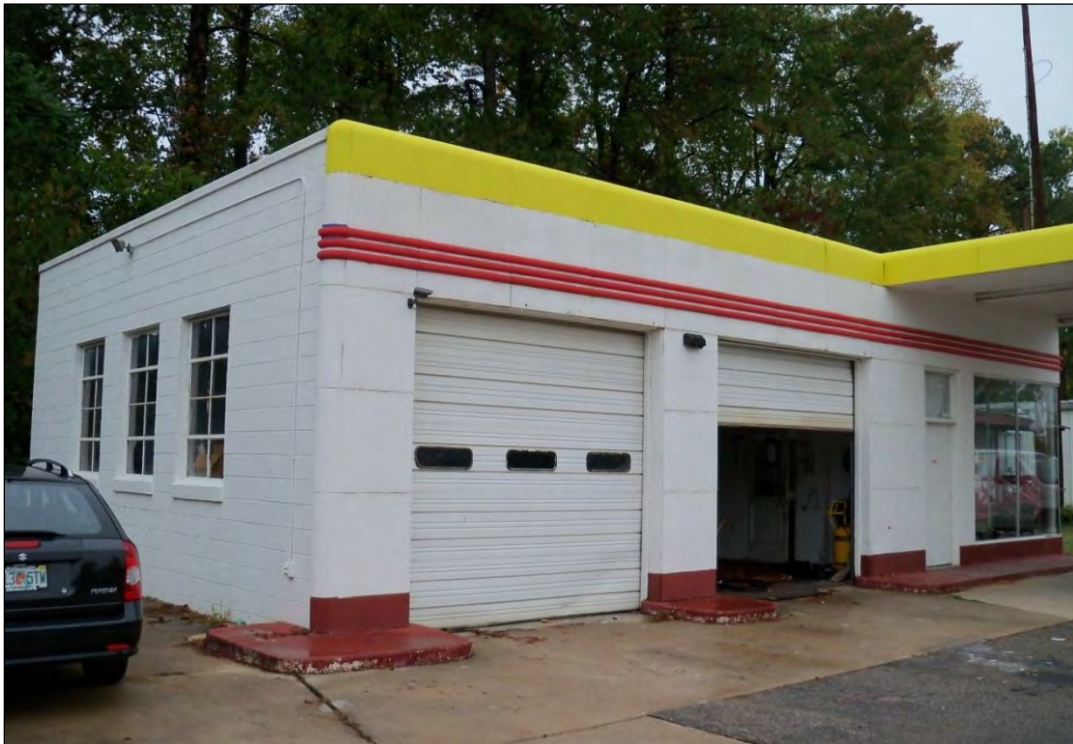
Photo 7: Southeast Oblique, Gulf Gas Station (WA 7363), With View of Distinctive “Gulf” Bands. Note the touch of the company’s trademark blue visible under the red paint.
